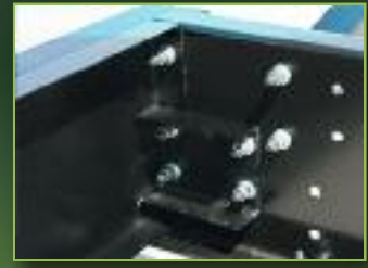
Epoxy and E-coated frame with Huck Bolt construction.
