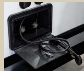
Standard outside shower provides both hot and cold water.
